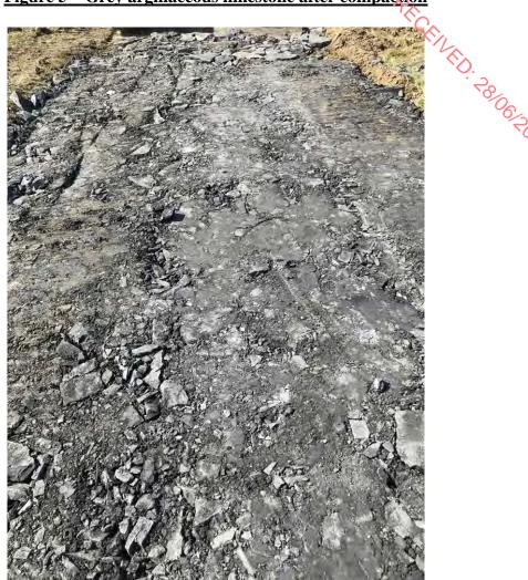
Figure 5 – Grey argillaceous limestone after compaction
